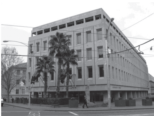
Figure 3. 55 St Andrews Place prior to upgrade (Source: Cundall, 2005)
