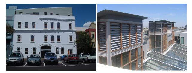
Fig C.8 Front façade and thermal chimneys of 60L Green Building (Source: ACF)
