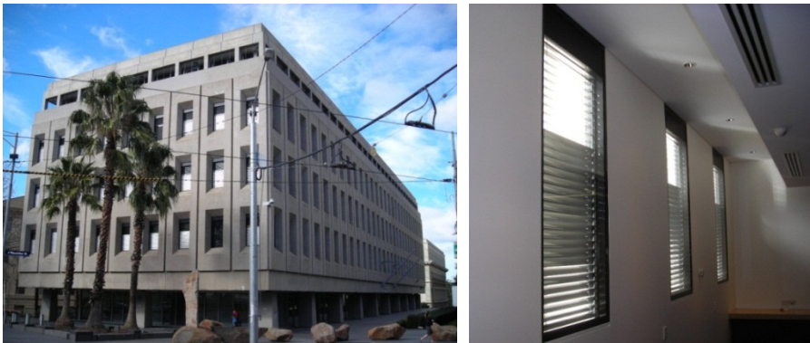
Fig H.20 55 St Andrews Place, Melbourne with external automated daylight guidance blinds (photos: author)
