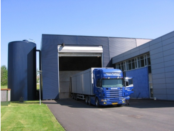
Fig 1.10 Wood chip delivery to district heating plant by articulated lorry (photo: author)
