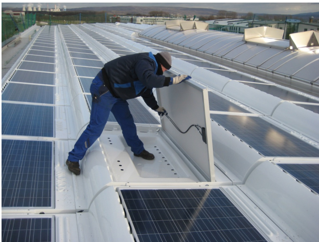
Fig I.5 PV laid on a flat roof. The system does not penetrate the waterproof membrane and also provides ventilation to the back of the panels. (Source: Solion)
